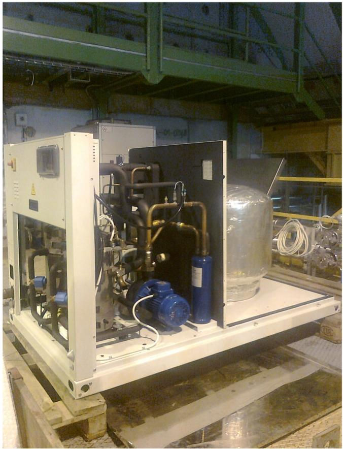
Consolidation of IT/TT cooling station: new plant installed
